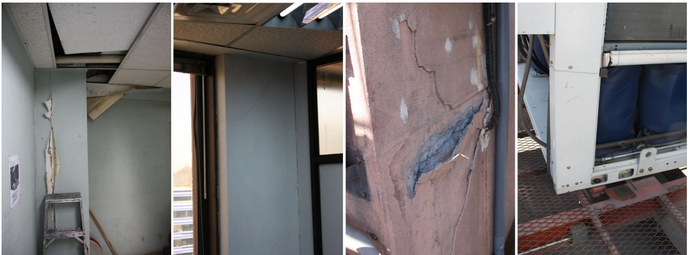
Fig.8 Observed damage after the 2010 Chile Earthquake
