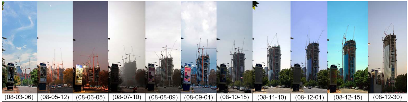
Figure 3. Construction sequence. Date (yy-mm-dd).
