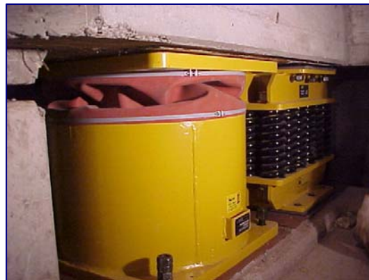
Figure 15 Viscous damper and springs bearing at the building's basement.
